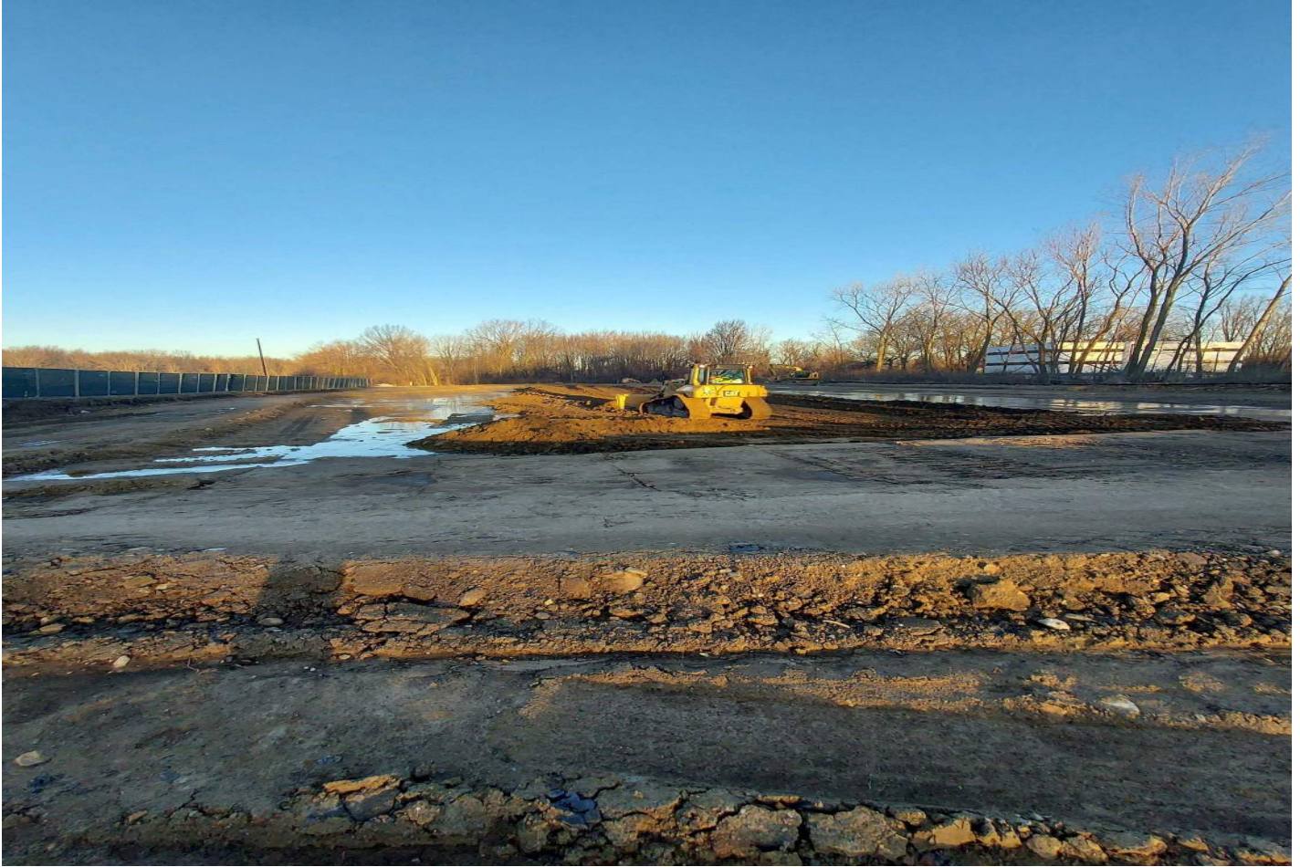
Cutting the unstable soil within the building pad
