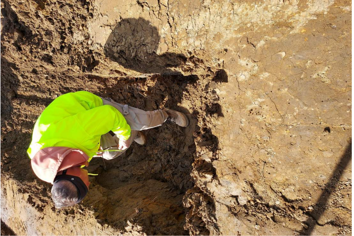
Depth check for bad area determined by proof roll
